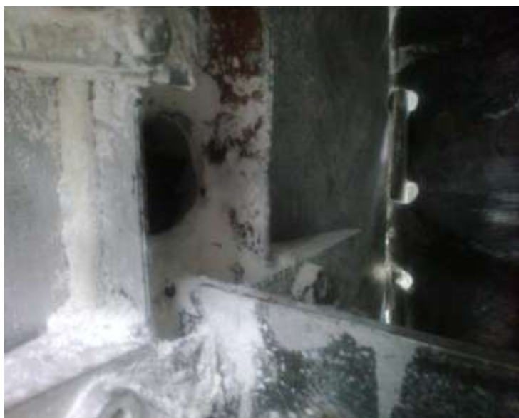
Fig. 3 – Holes on the Either Side of Machine
