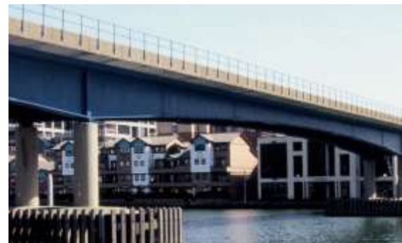
Fig: Docklands Light Rail Bridge, London, England.
