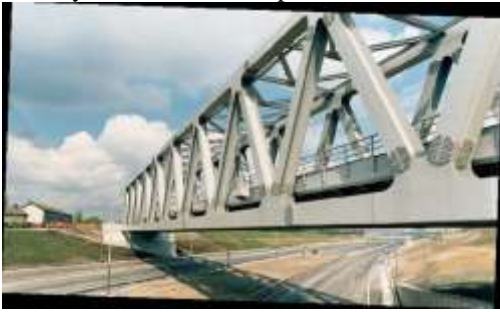
Fig: Brinnington Rail Bridge, Manchester, England
