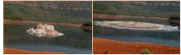
Figure 2 Lake tapping at koyna hydro project
