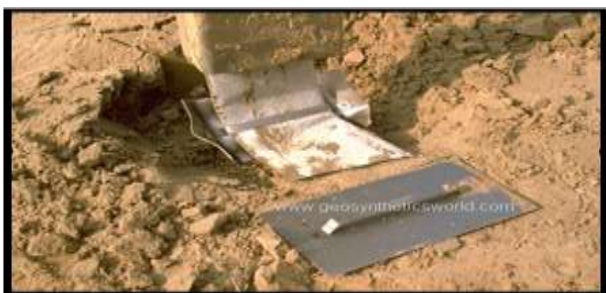
Fig.4.2.1 Insertion Of PVD
