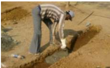
Fig. No. 3 Laying of P.C.C. bed
