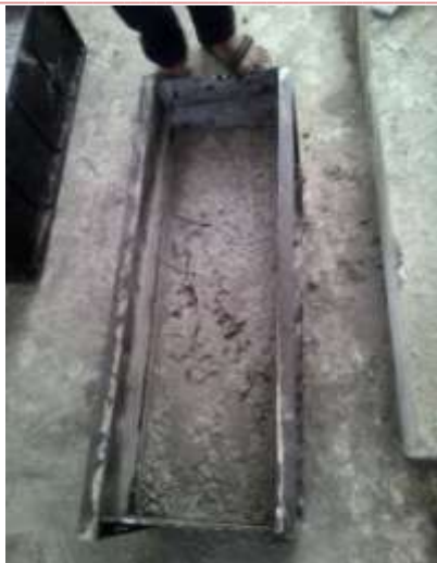
Fig.No.4 casting of column section
