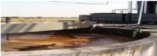
Fig.no. Oil and grease skimmer
