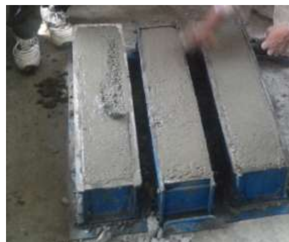
Fig.3 casting of beams
