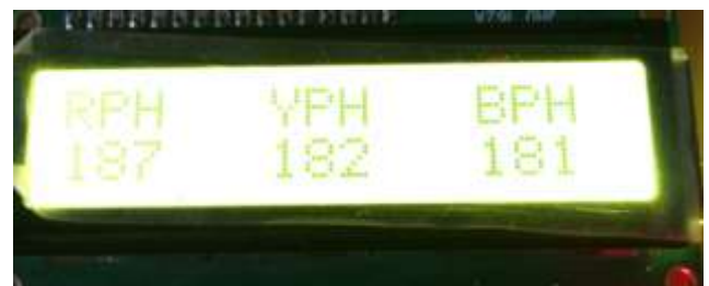
Figure 3: Under voltage display on LCD
