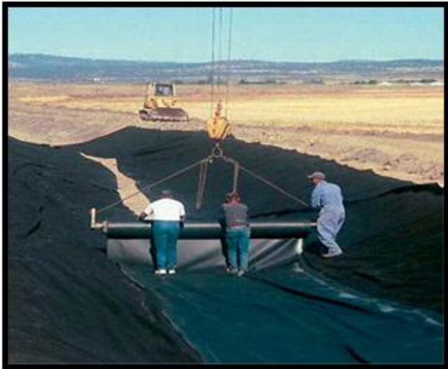
Fig. 4 BSE Type Reservoir Lining
