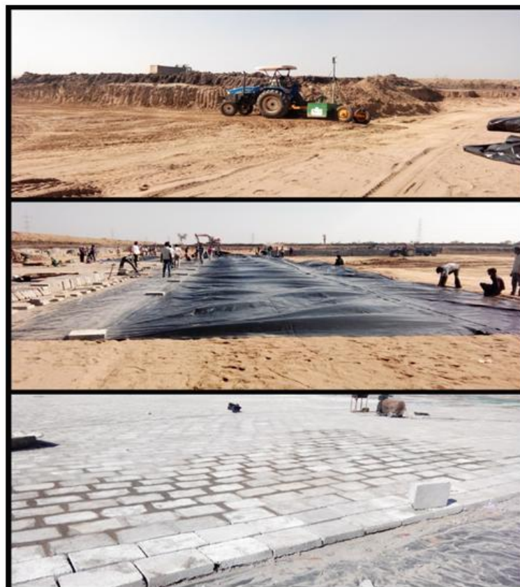
Fig. 3 Shp Type Reservoir Lining
