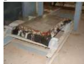
Fig.2.1 Rectangular steel frame with flexible PU membrane for casting the pre mould
