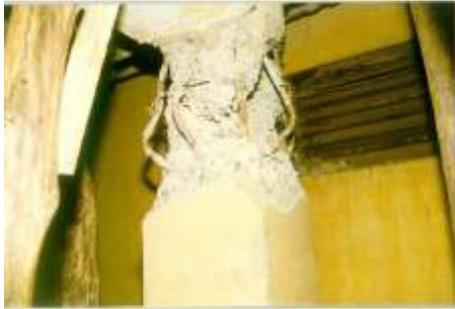
Fig-6 Damage to columns in Himgiri apartment.
