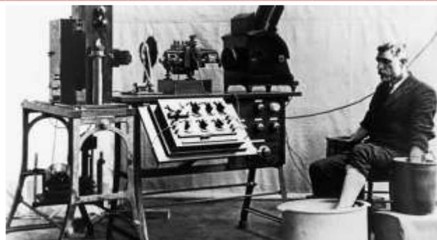
Figure 1. Old string galvanometer electrocardiograph showing the big machine with the patient rinsing his extremities in cylindrical electrodes filled with electrolyte solution..
